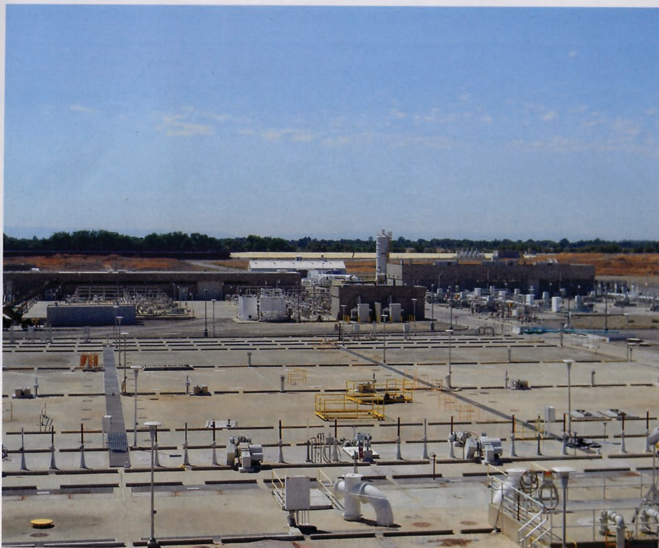
View of the high-purity oxygen activated sludge process from the Sacramento Regional Wastewater Treatment Plant control center. Joshua Nurmi
